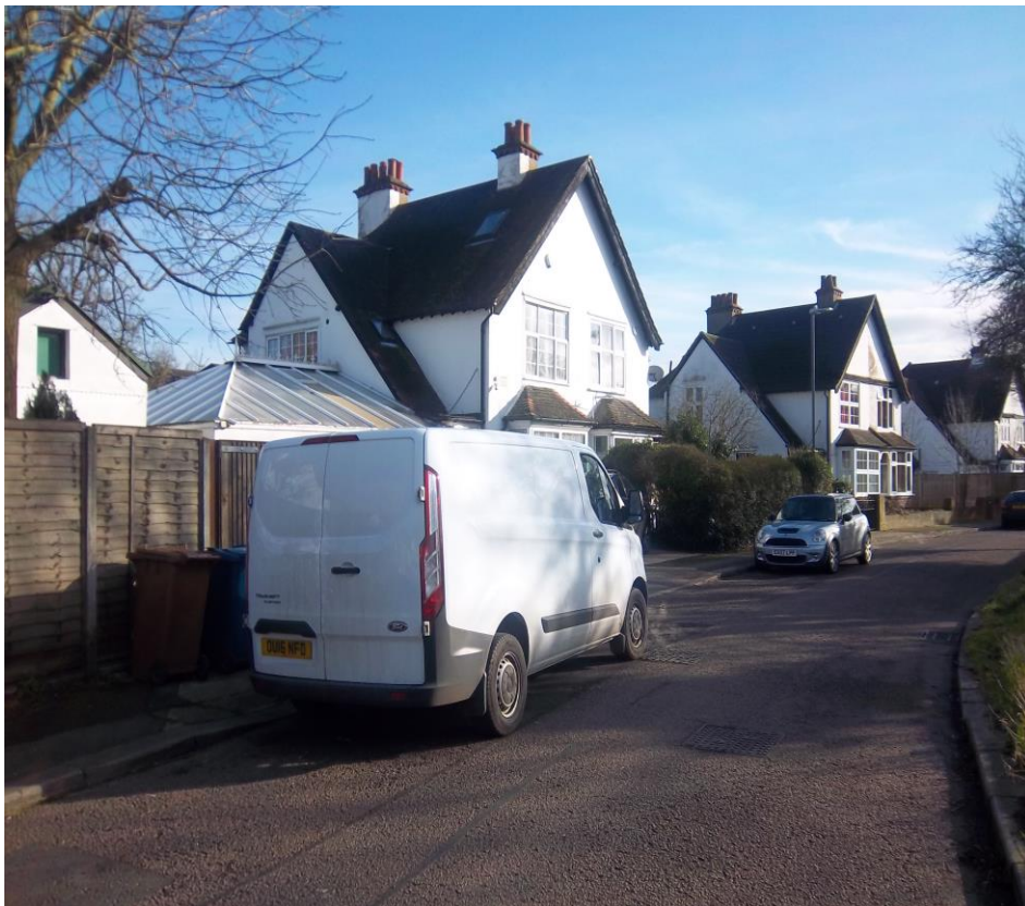
Side view and existing extensions
